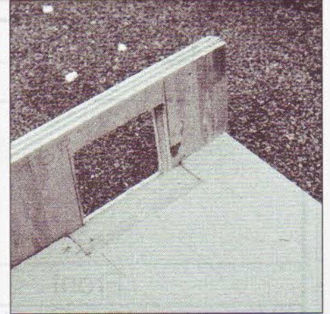
One end of the hinged baseboard showing the exit hole for the main line track. A piece of 9 mm thick ply is let into the insulation board base to provide a firm fixing for the track at this crucial position.
