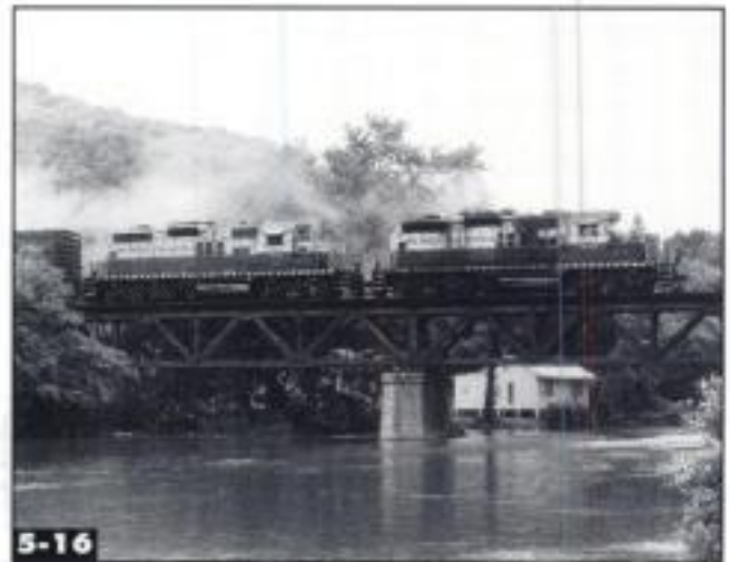
5-16 A pair of Warren deck trusses was used to span the Ramapo River on the New York, Susquehanna & Western. Don Darflinger
