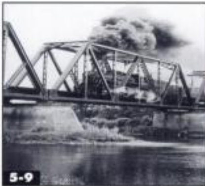
▲ Warren trusses, such as these Soo Line spans, are easy to identify, with diagonals in alternating directions in each panel.
