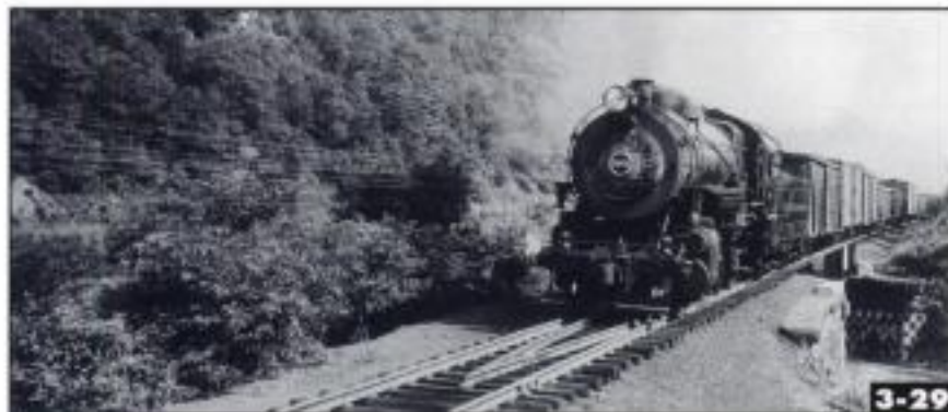
Guardrails typically extend 30' to 50' from the end of a bridge or trestle and usually come together at a frog. Norman Cooper
