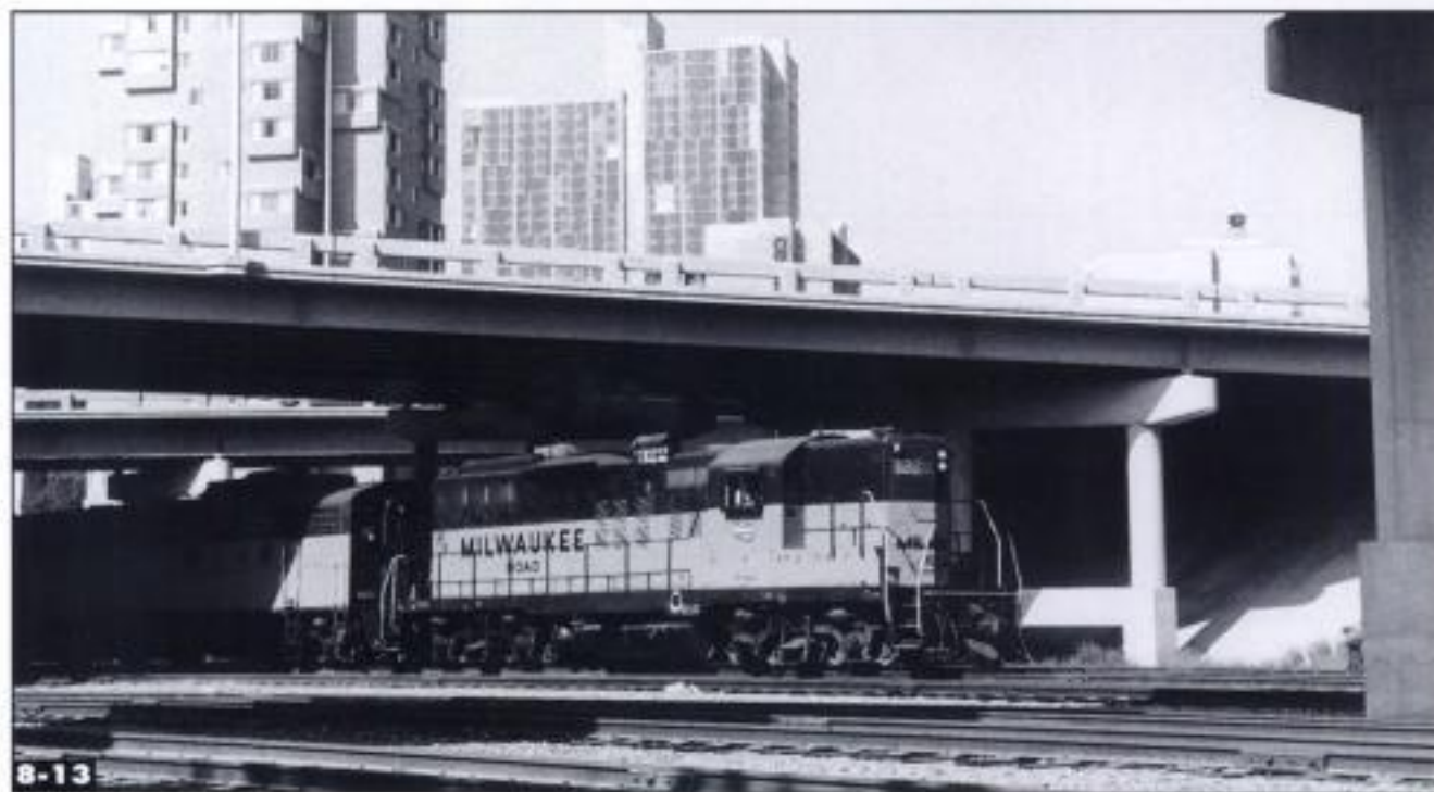
Many modern bridges use steel beams with concrete decks and railings and concrete piers of various designs. Stan Mailer
