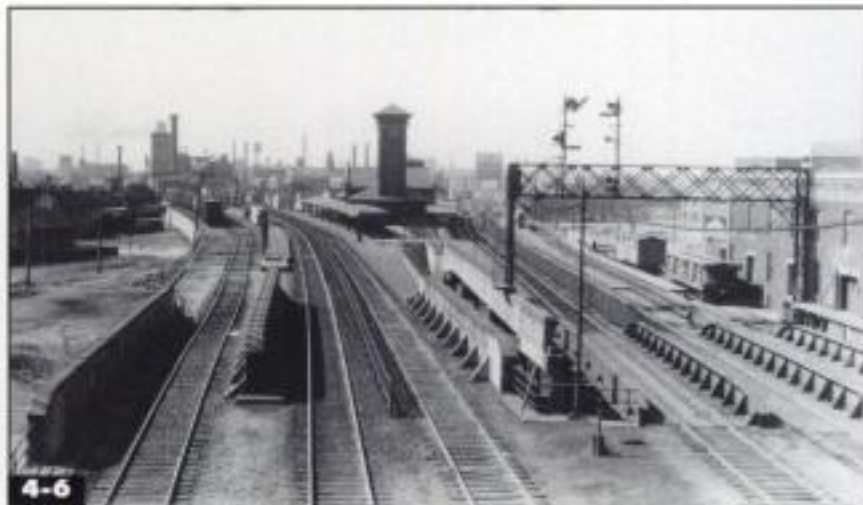
The three-track plate-girder bridge at left has a ballasted deck, while the three-track bridge at right is an open-deck that's been covered by metal plates. David P. Morgan Library collection
