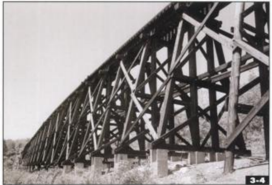
▲ Lightweight four-post trestles, like this 1860s structure on the Central Pacific, were common before the turn of the 20th century. D.L. Joslyn collection
