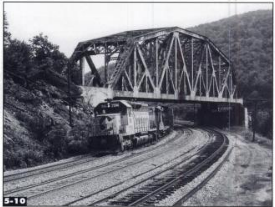
▲ Warren trusses, such as these Soo Line spans, are easy to identify, with diagonals in alternating directions in each panel.
