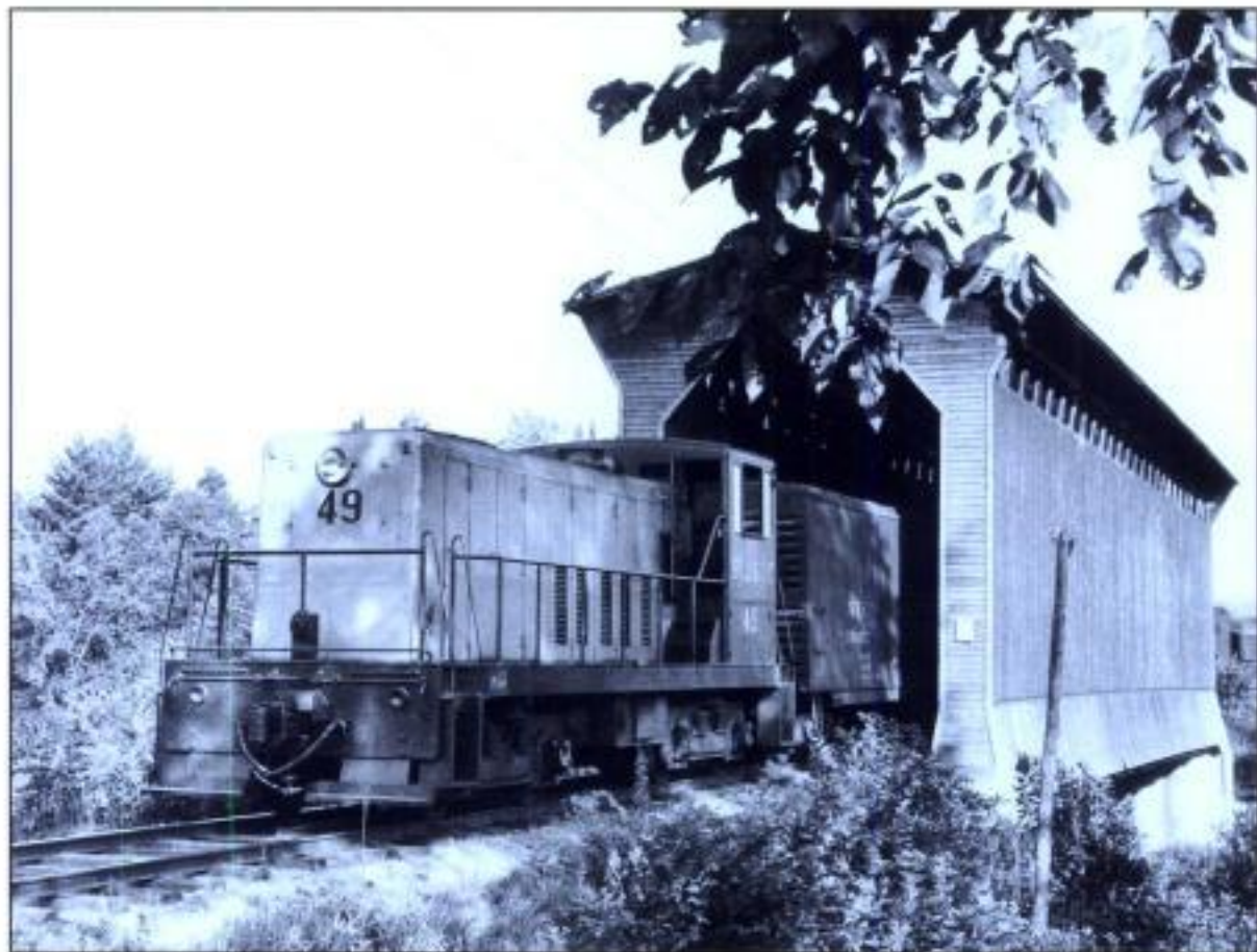
▲ Lurking under the sheathing of a covered wood bridge is a wood truss—a lattice in the case of this Boston & Maine structure. Richard Sanders Allen collection
