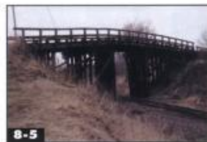
8-5 Some wood bridges used beams only, without king or queen posts. Jeff Wilson
