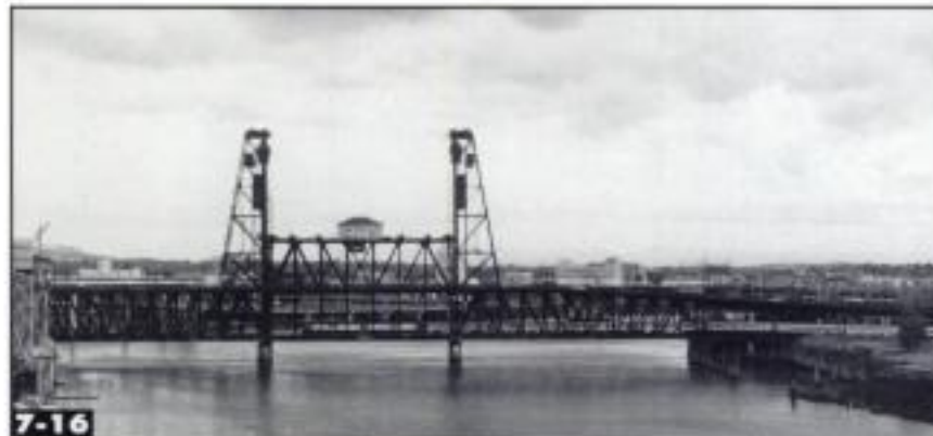
7-16 Portland's Steel Bridge is an example of a rail-highway lift span. The lower (rail) level can be lifted without disrupting highway traffic; the highway portion can also be raised for tall vessels. John C. Illman
