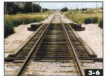
Note how the rails pass over the timber bulkheads at each end of this open-deck trestle. Jeff Wilson collection
