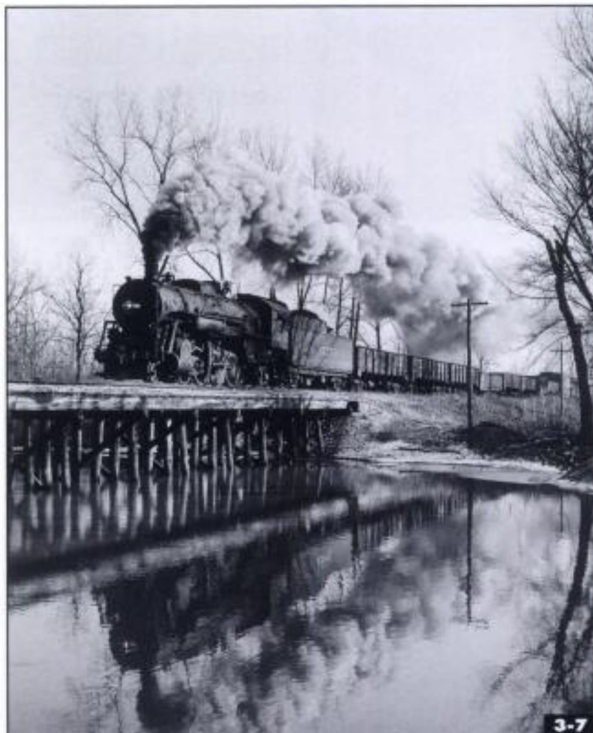
Look above the stringers and you'll see the ends of the planks that make up the deck of this ballasted-deck trestle. The rail and standard ties are visible on top of the ballast. J. Parker Lamb, Jr.
