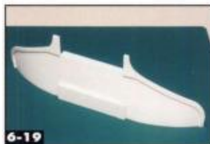
Here, the curved trim pieces have been installed, as have the .10"-thick base for the columns. Jeff Wilson
