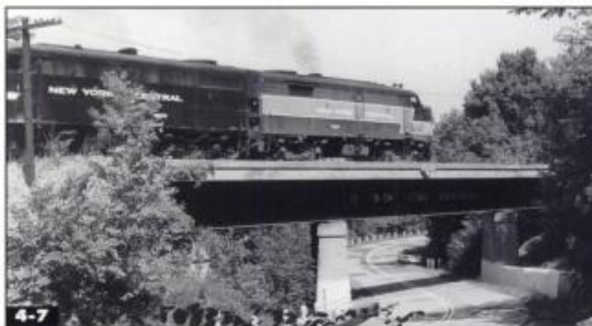
Ballasted deck girder bridges have a concrete trough atop the girders to hold the ballast and track. Jim Shaughnessy
