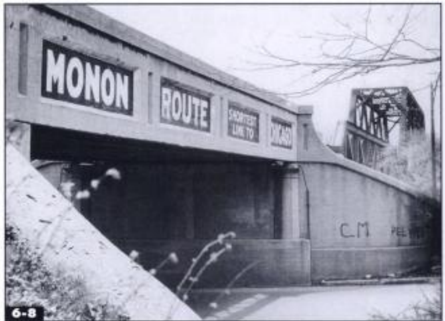
Many concrete bridges, such as this one on the Monon in Indianapolis, have interesting false facades and columns. Linn H. Westcott
