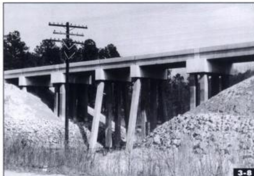
Concrete trestles replaced timber in many locations starting in the 1930s. G.E. Rashley
