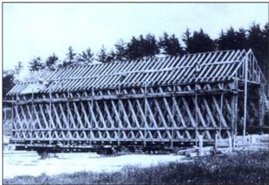
▲ Lurking under the sheathing of a covered wood bridge is a wood truss—a lattice in the case of this Boston & Maine structure. Richard Sanders Allen collection
