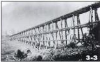
▲ Lightweight four-post trestles, like this 1860s structure on the Central Pacific, were common before the turn of the 20th century. D.L. Joslyn collection
