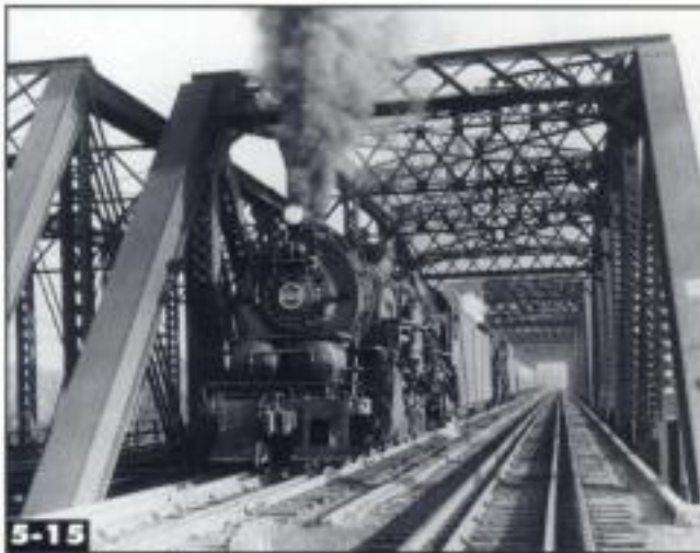
5-15 This double-track truss bridge on the Pennsy features a ballasted deck. The end posts are continuous-plate boxes, while the diagonals and hangers are double-laced. Don Wood
