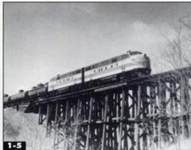
1-5 This wood pile trestle is on the Minneapolis & St. Louis near Oskaloosa, Iowa, in 1948. Trestles will be discussed in depth in Chapter 3. Robert H. Milner
