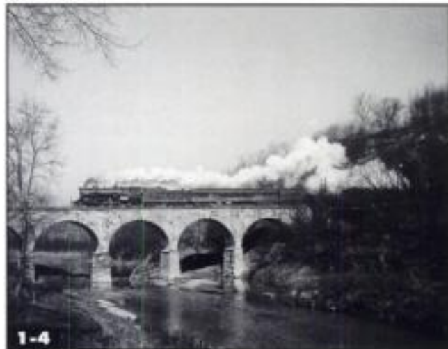
1-4 Many stone viaducts and bridges built in the 1800s were still in use well into the 20th century—some still serve even today. This Baltimore & Ohio viaduct is at Wheeling, West Virginia. J.J. Young, Jr.
