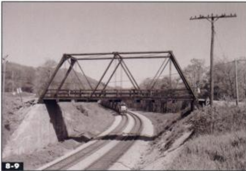
◀ An 81' iron Warren truss, this former railroad bridge was built in 1871 and converted into a road bridge in 1910. Historic American Engineering Record; Jeff Lowe
