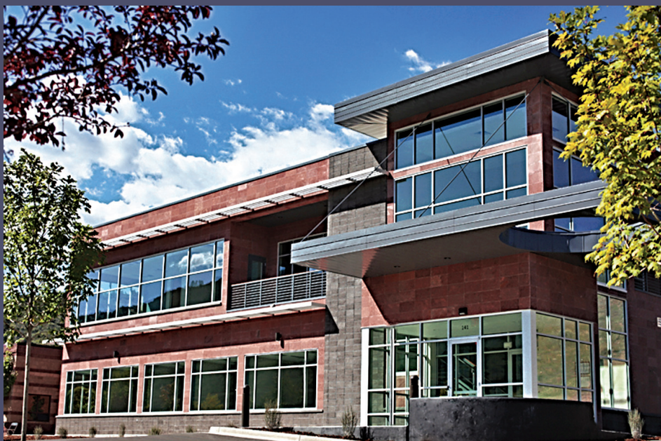
*Our manufacturing facility at 141 Burnett Drive, Durango, Colorado.
