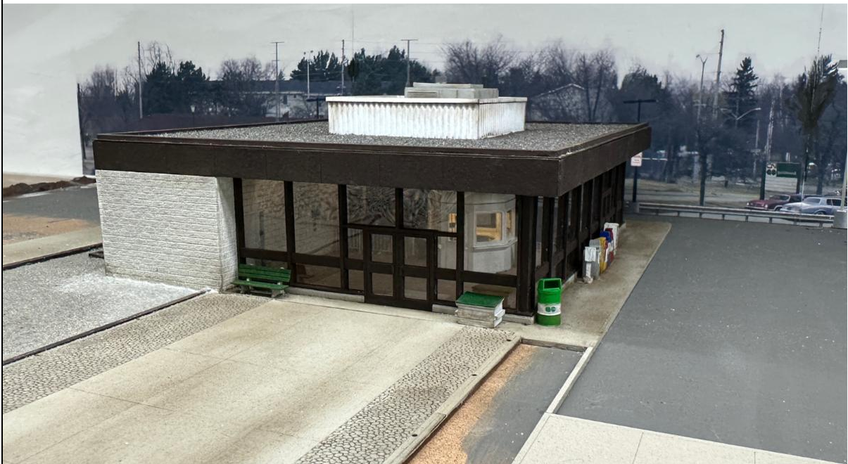
Guildwood Station, seen under construction earlier this week, is one of the "bland" steel and concrete stations Jason is scratchbuilding for his layout.
