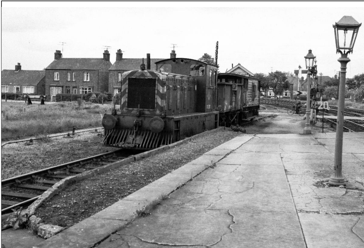
1. D2201 brings a short train into Wisbech East station from the March end. This platform served W&U trains (the trackbed was raised to make accessing the coaches easier) with March-Magdalen Road trains using the two platforms to the right. The buffer stop on the left is on one of the W&U sidings, with the former depot area just out of shot. on the left. The signalbox box still proclaims Wisbech Station – it was not named Wisbech East until 1948.
