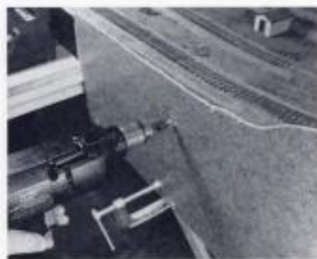
ABOVE: Use a countersink drill bit to set the screws for the fascia below the surface. Use C-clamps to hold the panel in place while you drill the holes. After the screw holes are filled, sanded, and painted, they will be invisible. RIGHT: Pieces of 1 x 1 molding work well for fastening the fascia corners together. These pieces can be used both above and below the table surface as needed. Be sure to drill pilot holes for the screws, as these small pieces of wood will split easily.
